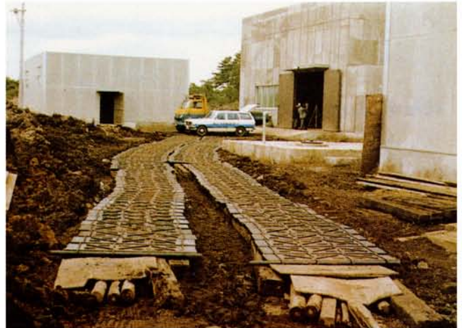
加速器実験室への搬入路（泥道をキャタピラにて補強） Access to an experimental hall (the muddy road is kept passable by a pair of "caterpillar treads.")
