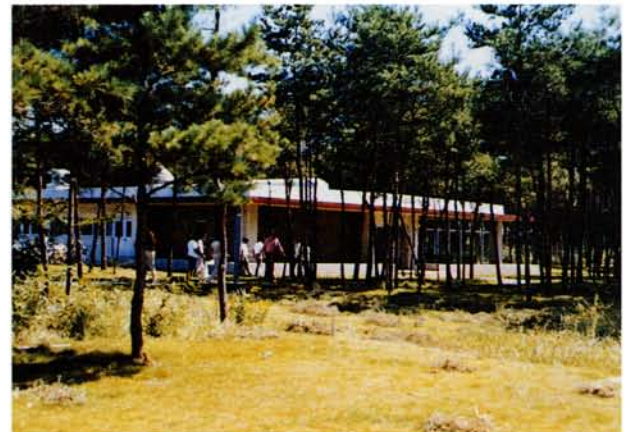
職員食堂 Completion of the Cafeteria.
