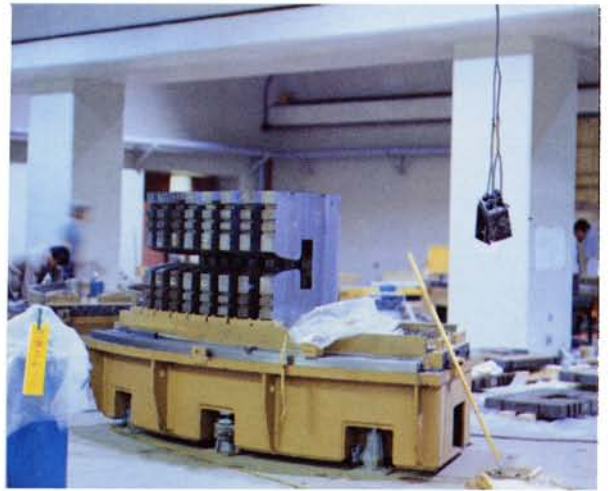
ブースター電磁石組立開始 Installation of the Booster magnets is started.
